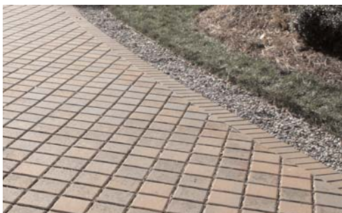
This innovative pavement creates an upscale look for driveways; it also helps builders comply with local stormwater regulations.
